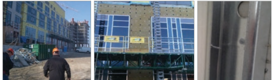
Exterior walls - Insulation to steel stud
