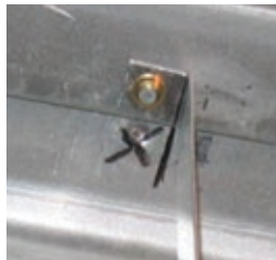
M034 fastener used to hang HVAC Duct Strap
