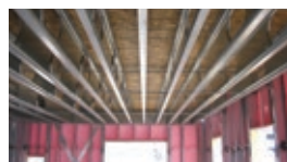
OSB and plywood to iSPAN joists
