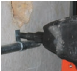
12HSMPO34 clip assembly used to secure conduit
