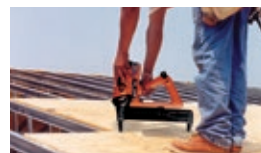
Plywood attachment—using TrakFast plywood to steel pin
